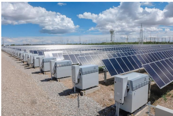
Figure 2: Energy storage in a solar farm
