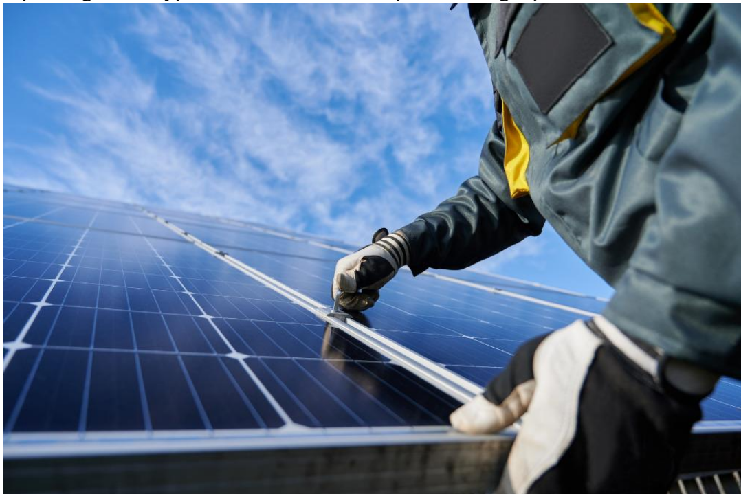
Figure 4 Repair of solar panels ( https://sistinesolar.com/solar-panel-repair-services/ )
